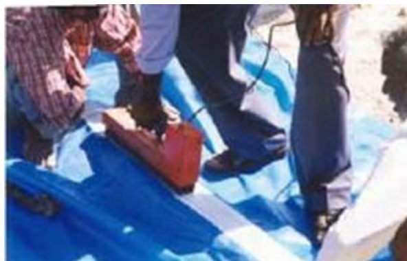
Plate 3: Heat Sealing of LDEP Sheets
