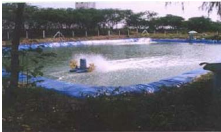
Plate 1: Earthen Pond Lined with 250 gsm LDPE Sheet
