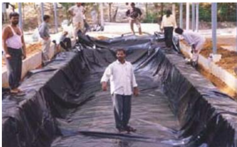
Plate 2: Laying of 700 gsm Synthetic Fibre Sheet in a Raceways Tank
