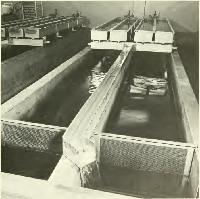
FIGURE 19. Rectangular aluminum troughs (background) and concrete tanks. Small swim-up fry generally are started on feed in the troughs and then transferred to the tanks when they are 1\frac{1}{2} -inch fingerlings. (FWS photo.)
