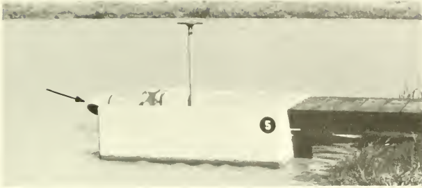
FIGURE 22. A pond catch basin should have a supply line (arrow) to provide fresh water to the fish when they are collected in the basin. This pond outlet also has a valve to open the pond drain.
