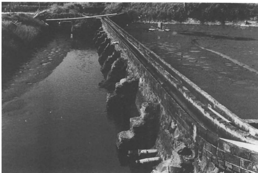
Figure 2. Old style concrete pond wall in Taiwan with double water supply canal on top. Photograph from Fast et al. (1989).
