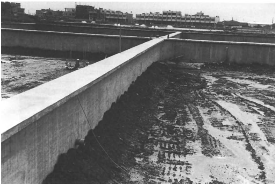
Figure 3. New style reinforced concrete pond wall under construction in Taiwan. Photograph from Fast et al. (1989).
