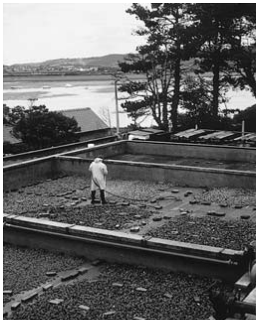
Fig. 12.1 Conwy mussel purification tanks.
